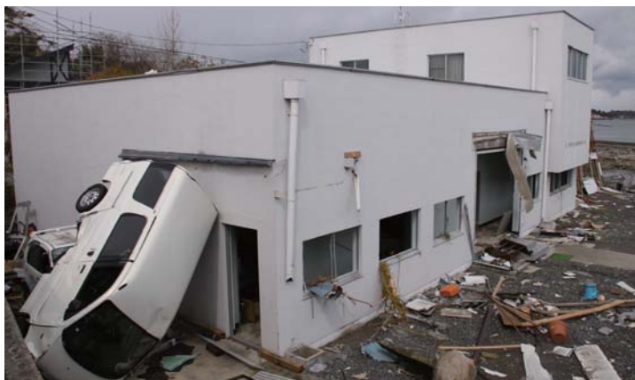
Tsunami attacked even Shelter that is 12 meters above sea level
