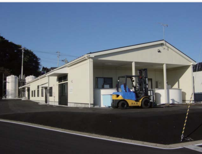
1 Shared seaweed processing and treatment facility
